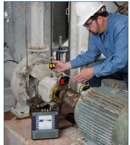
*Emerson's CSI 2140 now interfaces with leading laser alignment fixtures for a single-box solution for your route-based predictive maintenance program.*
